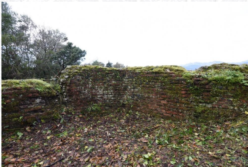
Unutrašnja strana zidana u opeci / The inner side built in brick
