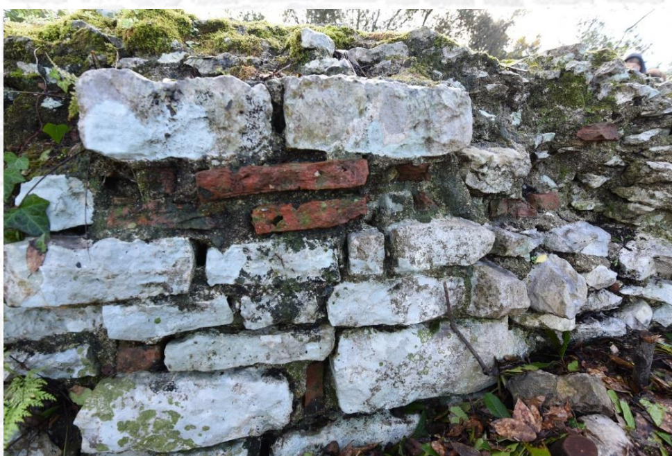
Detalj zidanja spoljašnjeg zida / The detail of building the outer wall
